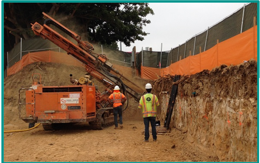
Soil Nail Wall Start of Construction
