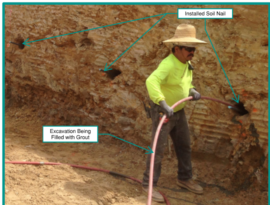
Soil Nail Wall installation
