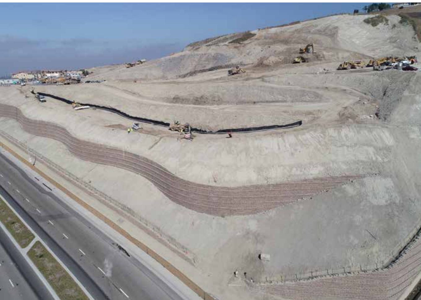
Figure 5. Construction of a three-tiered MSE wall/slope combination (foreground) and ongoing buttress excavation (background). (Photo courtesy of John Carter.)
