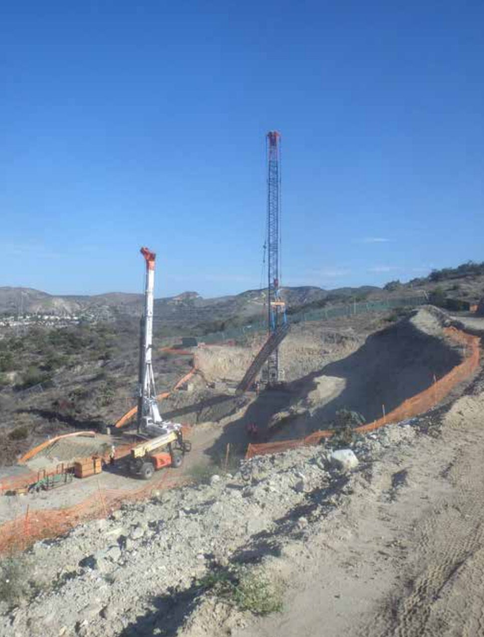
Figure 2. Shear pin construction along the northern boundary of Portola Northwest, adjacent to Whiting Ranch Wilderness Park.
