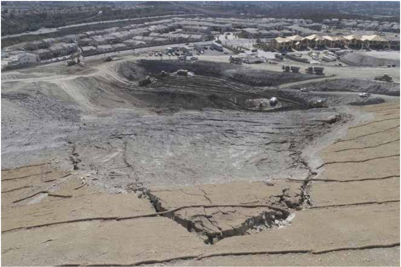
Figure 3. A typical day of buttress grading... another backcut failure along a remolded clay seam during buttress grading on Portola Northeast. (Photo courtesy of John Carter.)
