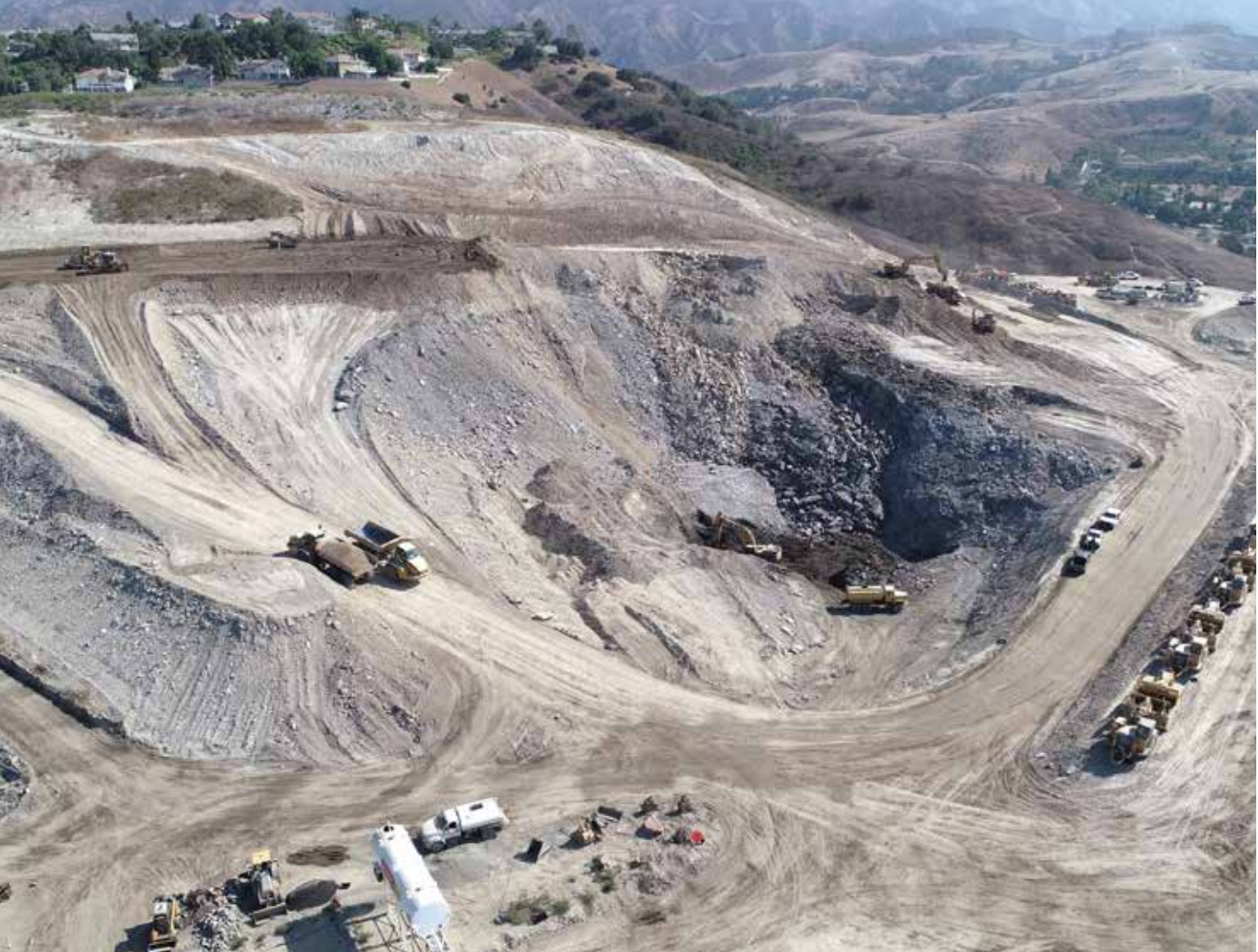
Figure 4. Slot-cutting to reach keyway elevations. Benching and placement of fill in the recently completed slot behind the water truck (foreground). Collapse of excavation sidewall along a remolded clay seam daylighted in the next keyway slot (background). (Photo courtesy of John Carter.)
