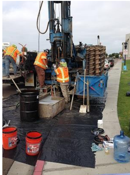
Mud Rotary Drilling at the San Diego Convention Center
