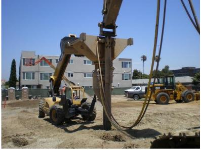
Stone Columns Being Installed in San Diego, California
