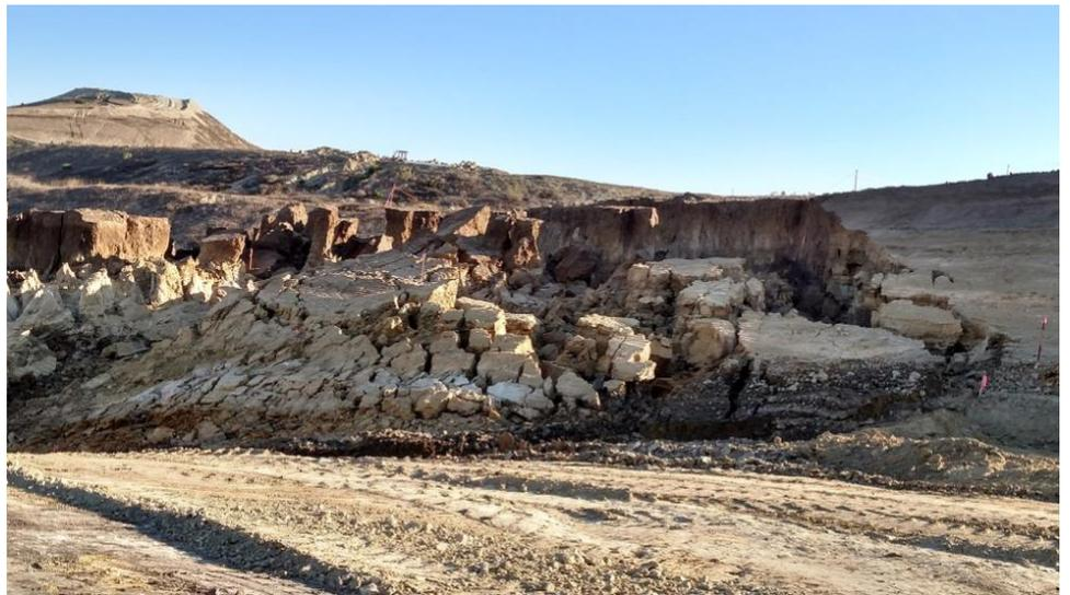
*Grading Temporary Backcut Failure in Lake Forest, California*
