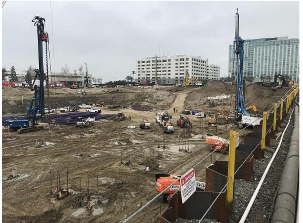
*Sheet Piles and Auger Piles for Pacific Gateway in San Diego, California.*
